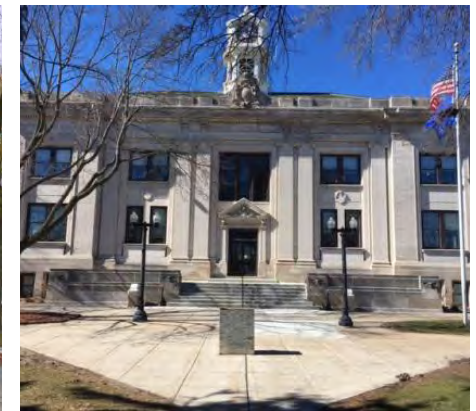
Sauk County Courthouse
