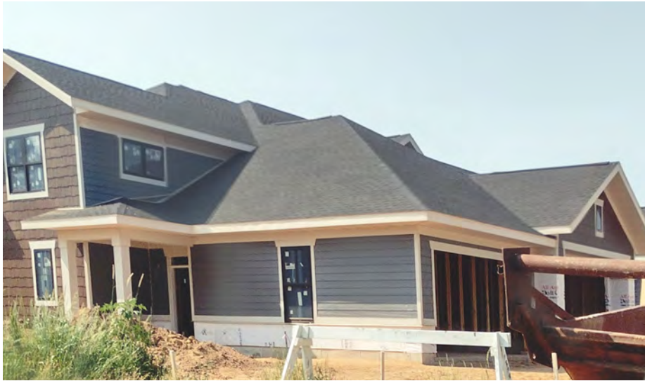
Construction of new single family homes
