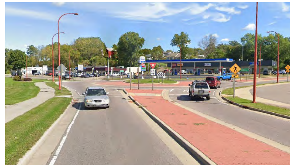
Roundabouts in Baraboo provide access for multiple modes of transportation.
