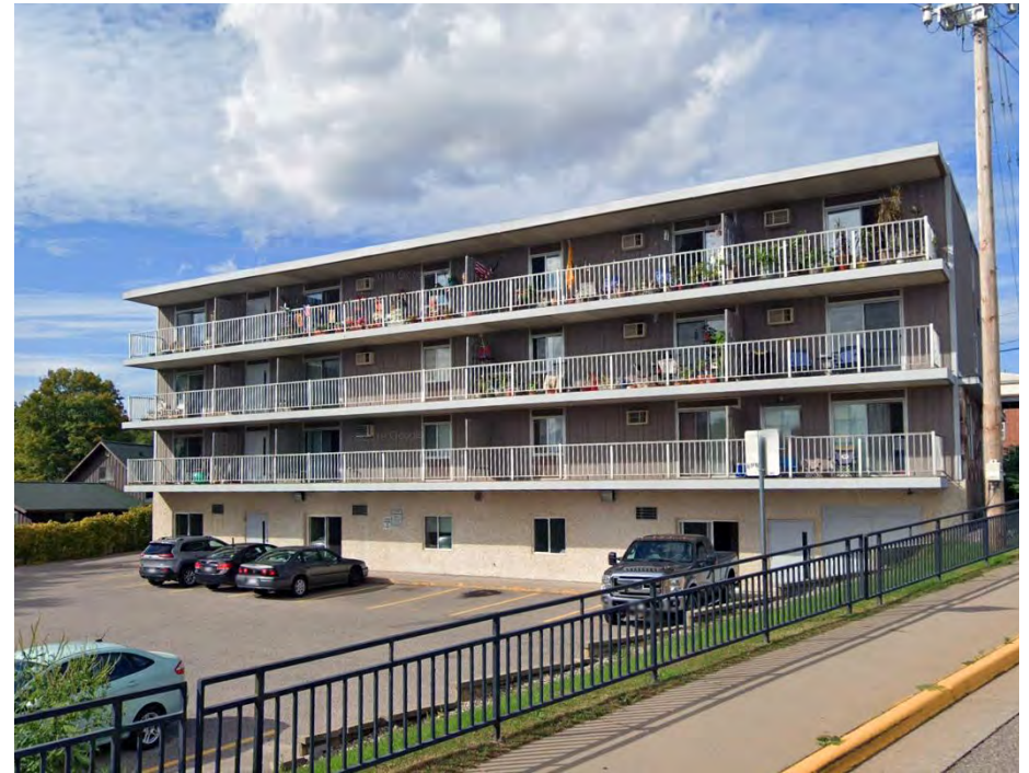
Riverview Tower Apartments
